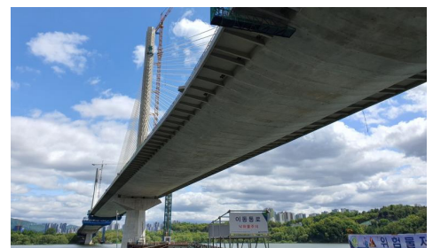
(b) Girder construction at Godeok bridge
