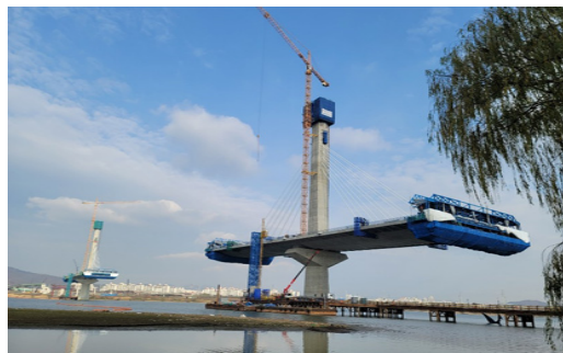
Fig. 16. Construction of pylon and girder
