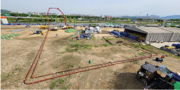
Fig. 17. Pipe pressure test of C80
