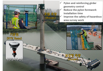
Fig. 28. Application of high-precision GPS
