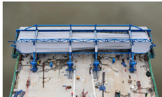
Fig. 20. Installation of retractable form traveler shelter
